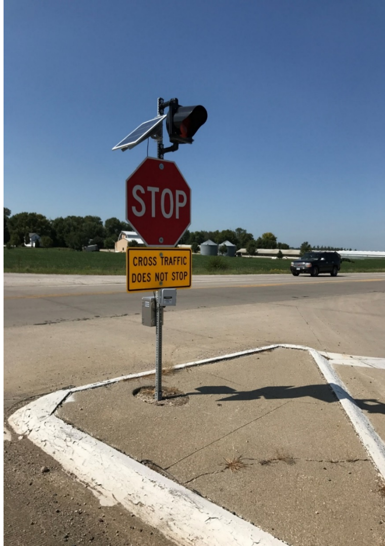
Figure 7: Flashing Beacon Installation
